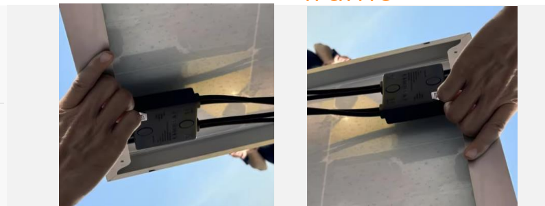
Mounting optimizer with PV panel frame
